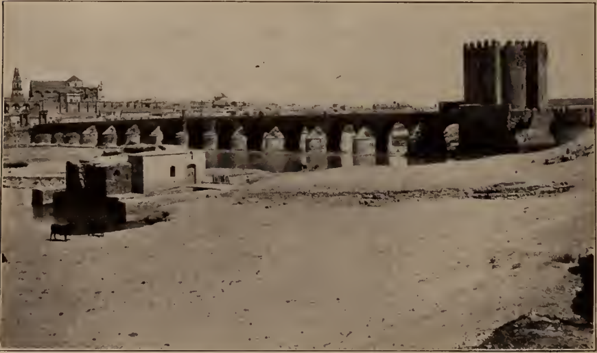
THE OLD BRIDGE AT CORDOVA.
